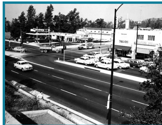
Late 1950's Multi-Lane Pavement
