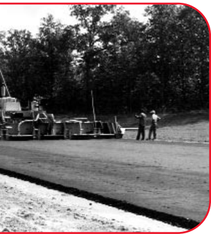
This is a Blaw-Knox PF-220 paver from the 1960's. Note the width of the paver—using screed extensions. It appears to be about 30 feet wide.
