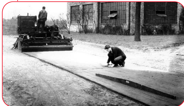
This is testing a 10-foot wide Barber-Greene machine in 1935. The young engineer monitoring the work is H. Ashley Barber.
