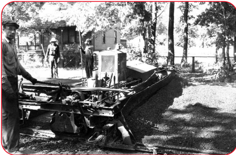
An automated screed. This one required a rail or form to ride on. This is a job in Michigan in 1934.
