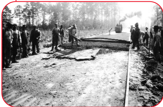
A hand-operated screed being used on a job in the 1920's.
