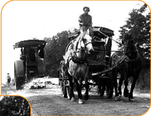
A water distributor on a macadam road operation in Maryland in 1913.
