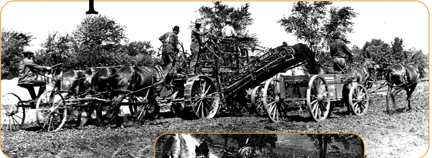
This Russell elevator-grader probably operated some time between 1910 and 1920. There were eight horses or mules in front and four in the rear. Notice the rear drop-dump wagon.
