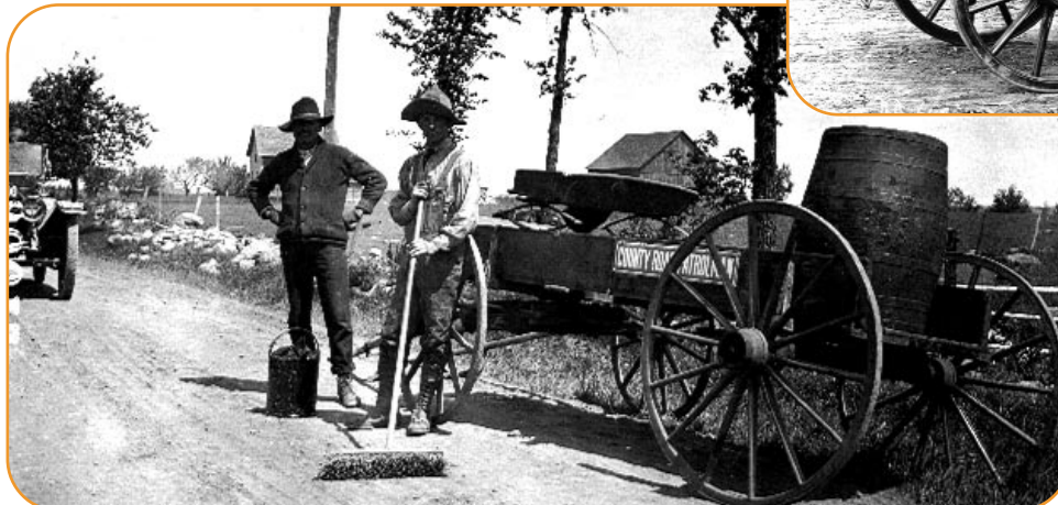
Wooden barrel of asphalt and a pour-pot used for maintenance around 1915.
