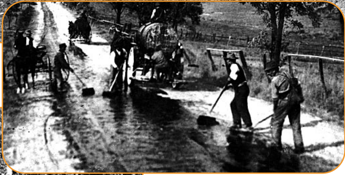
Another road oiling operation.
