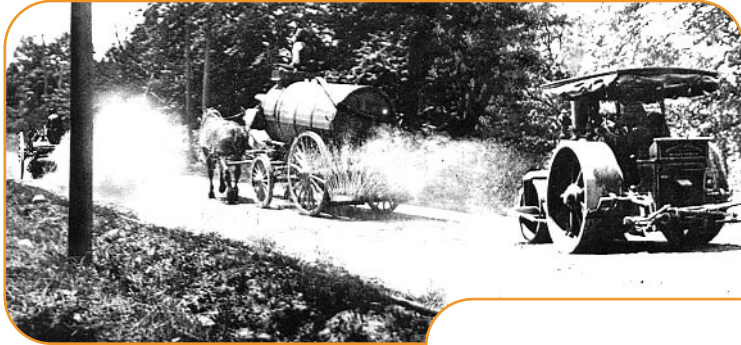
Early road-oiling operation some time between 1900 and 1910. The horse-drawn broom is in front, followed by the water distributor, then the roller towing the asphalt distributor.
