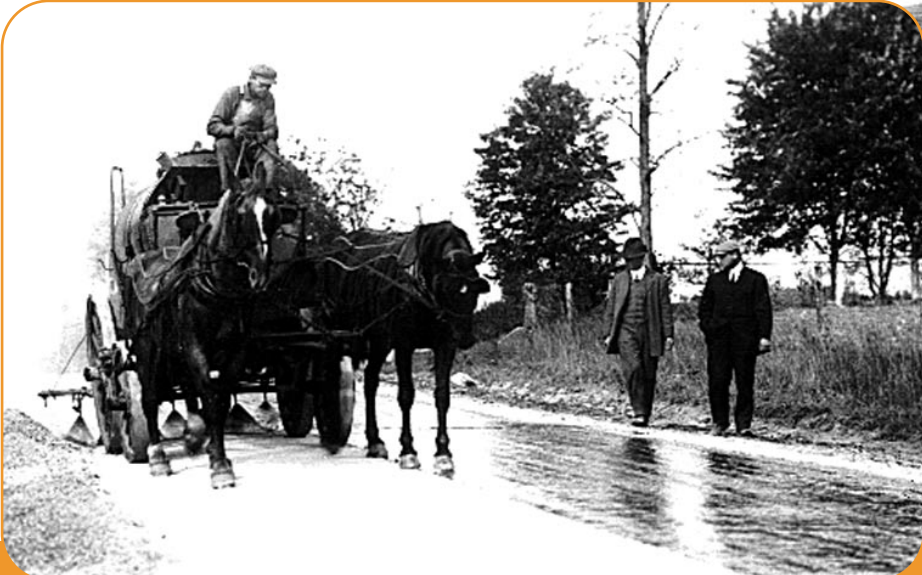
A horse-drawn asphalt distributor around 1910. The gentleman on the far right is Herbert Spencer, Asphalt Institute President from 1941 to 1947.
