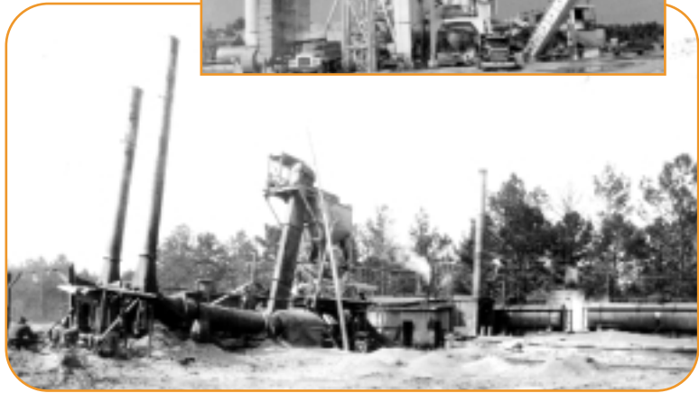
A circa 1910s asphalt plant.
