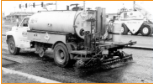
Above: Circa 1910 asphalt distributor. Note the solid rubber wheels.
